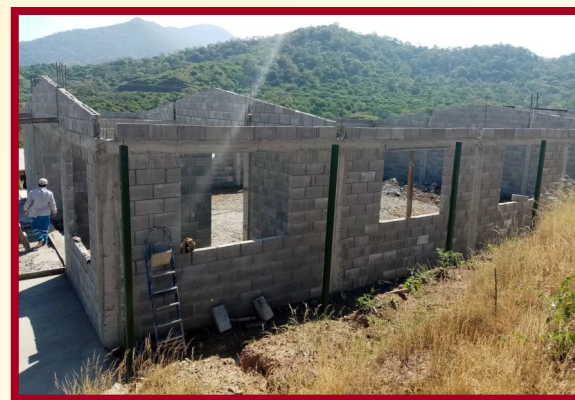
New church construction in Peru.
